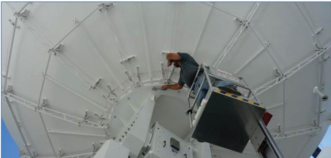
*EEC Defender S850 S-Band Antenna/Pedestal Assembly Installation*
